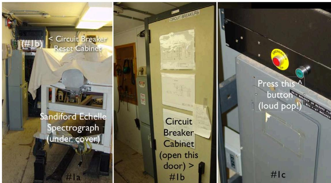
**Figure 5.** Cass Echelle storage room by north pier on the third floor. Reset breaker location.
